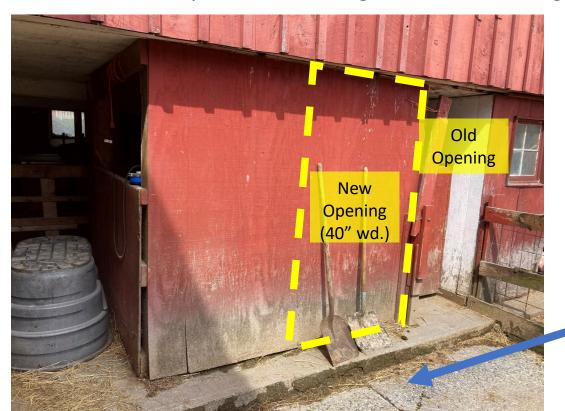
Cut new opening in plywood partition wall and close off the old opening.
